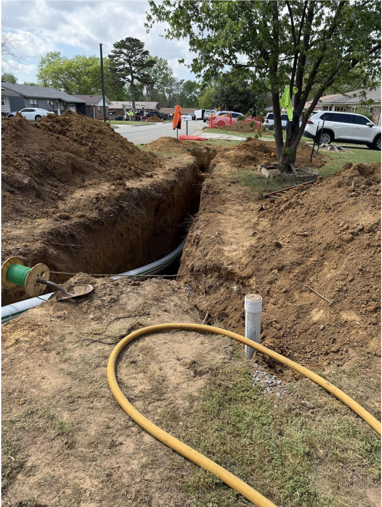
HDPE Pipe with Tracer Wire and Service Cleanout
