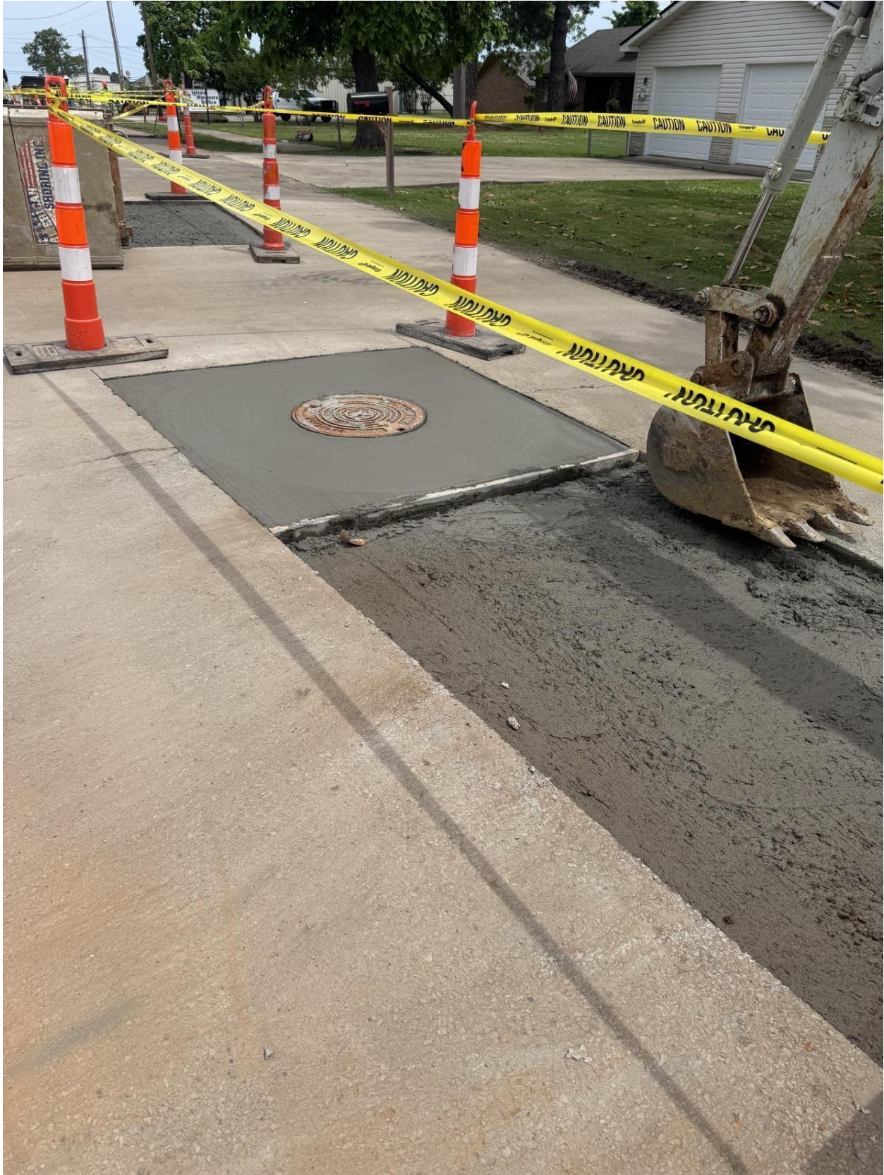
Manhole Concrete Cap and Asphalt Deep Patch
