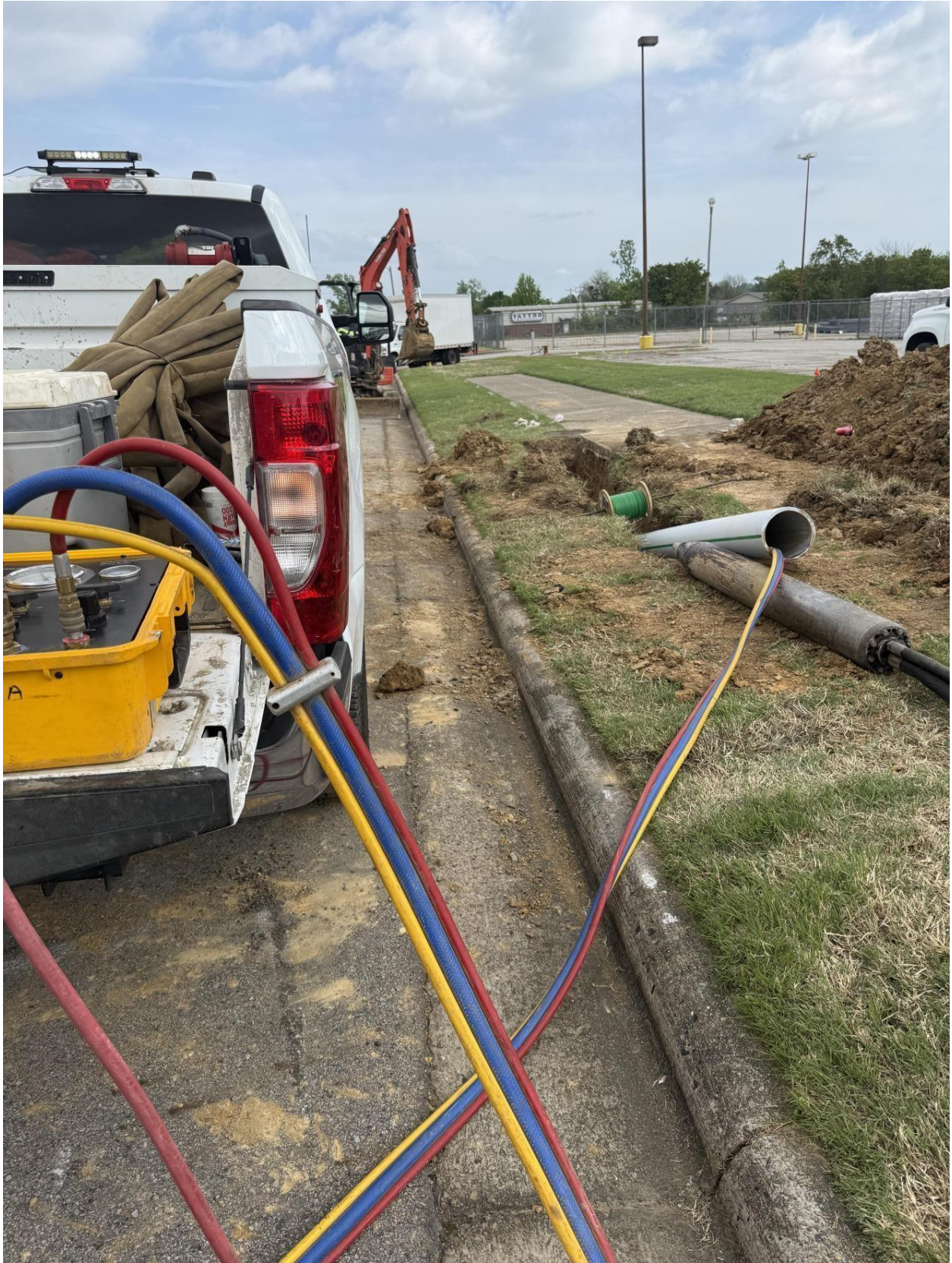
Bursting Head and HDPE Pipe following Pipe Burst
